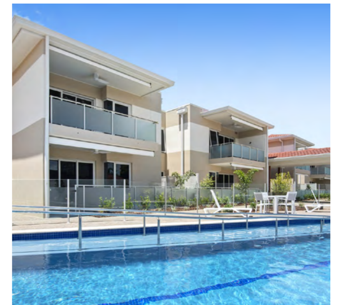
New Apartments Block B now under construction.
